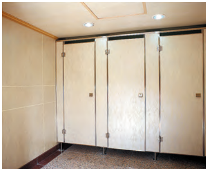
· 浴廁搗擺 Door panel of bathroom
